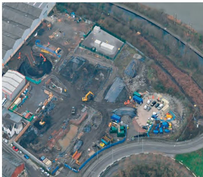
Neath site during works
