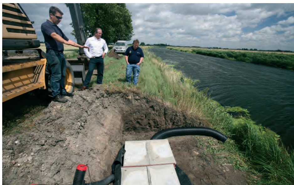
Otter Holt construction
