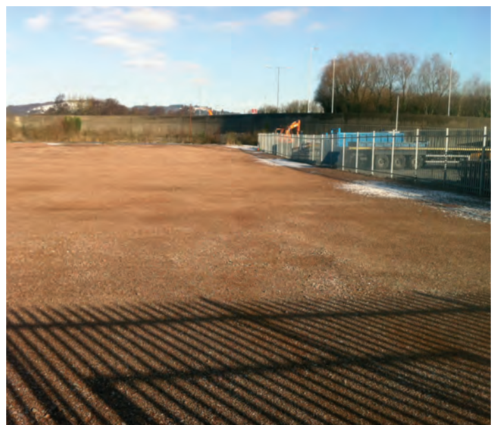
Neath site after works were completed
