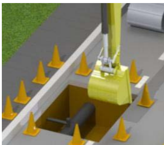
Figure 7 Service Connection Excavation
