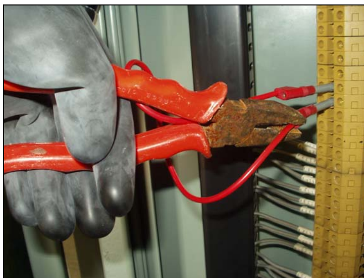
Figure 40 – Safe Application of Short Circuit
