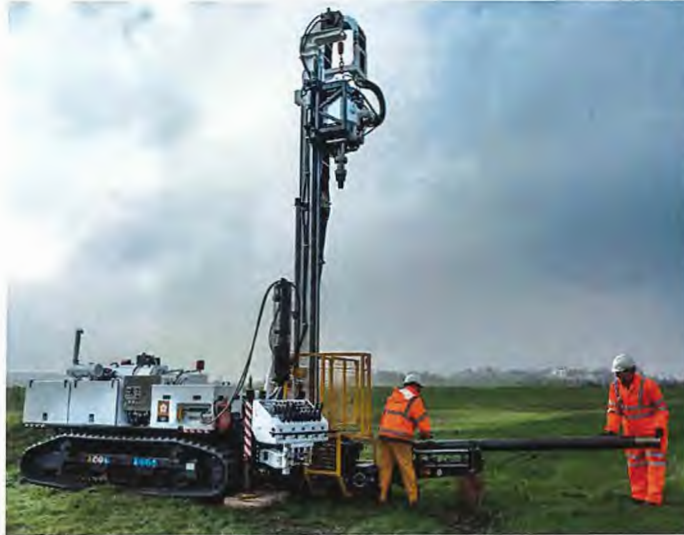
Figure 3.1. - Example of a Sonic Drill Rig
