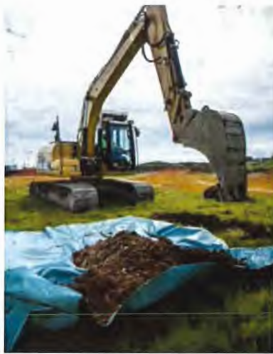
Figure 3.2. -14 Tonne Tracked Excavator
