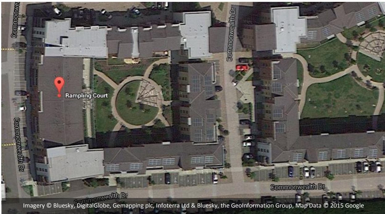
Figure 16 – PV panels at Rampling Court
