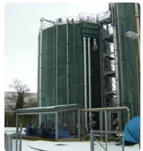
Anaerobic digesters at Didcot Sewerage Works
